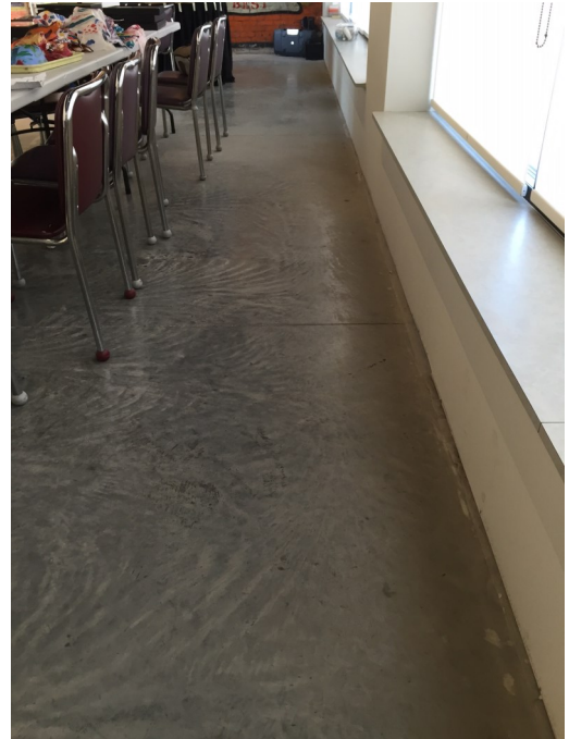
Concrete slab floor
